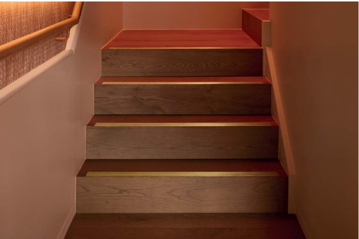
Nosings with brass inlays offer a durable, high-contrast edge detail and are often used in commercial fit-outs where visibility and compliance are key.
